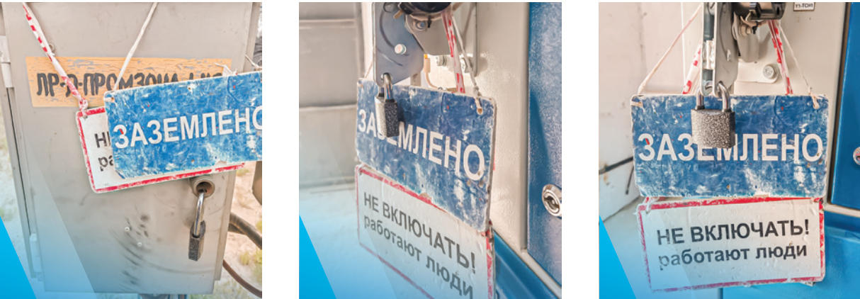
MREC: implementation of Lock Out - Tag Out (LOTO)
